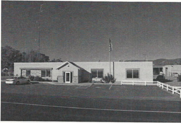
Raft Rural Electric Co-op 2010
